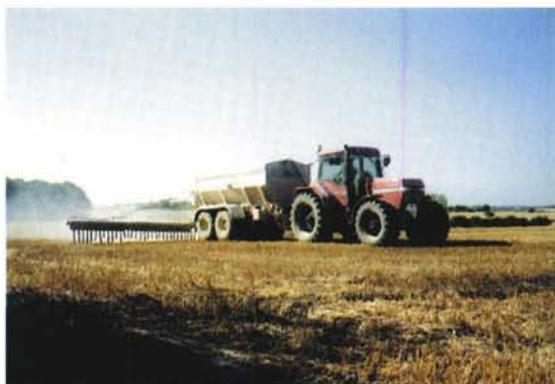
Photo 1.2 – Épandage de chaux pulvérulente [F.X. Gaumont, MEAC]
