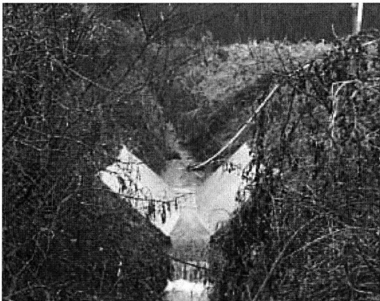
*Fig. n° 2 : Pre-formed flume structure imbedded in the ditch at site A1*
