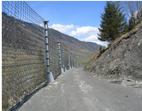
Figure.2. Typical situation for a system with fixed rotation next to a road for forestall work and the object of protection more down-slope
