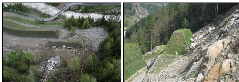
Figure 1. Example of reinforced soil embankment used for rockfall protection in Cogne (Italy)
