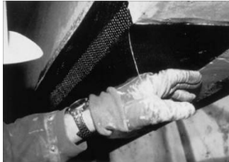
Figure 5. Beam retrofitting with FRP bonding on lower side.
