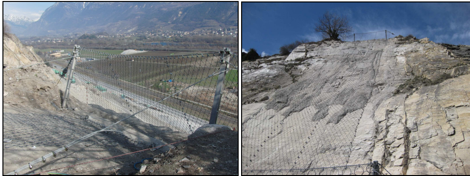
Figure.2. (left) impact zone at the top and (right) 40 m tail drapery
