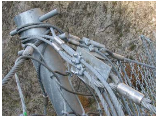
Figure.2. GTS braking system working by friction
