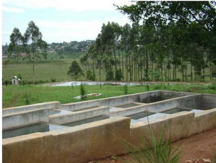
Tannery treated effluent discharges into the Nabajjuzi wetland (photo: P. Isagara)
