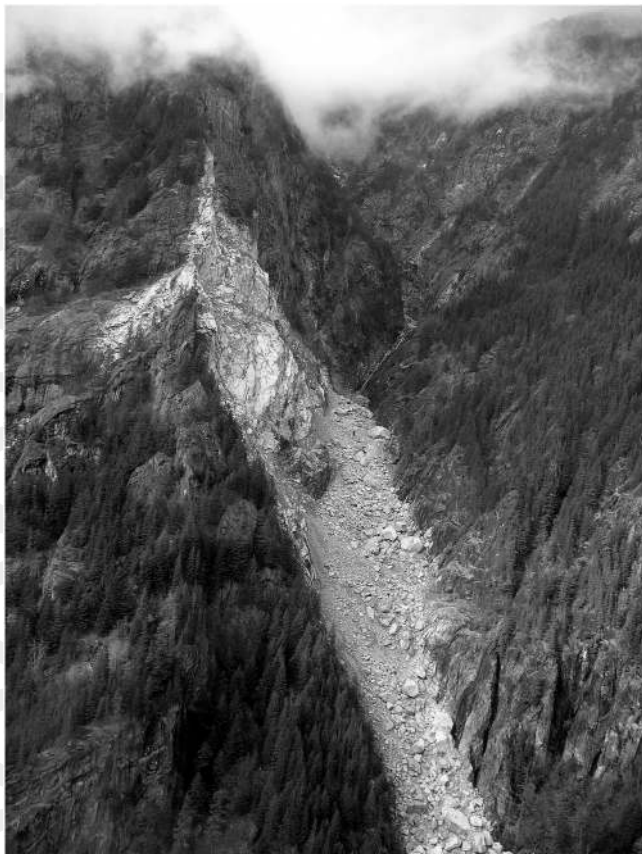
Figure 3. An aerial view of the source and part of the deposit of a small rock mass fall back analysed by Strouth and Eberhardt (2009).
