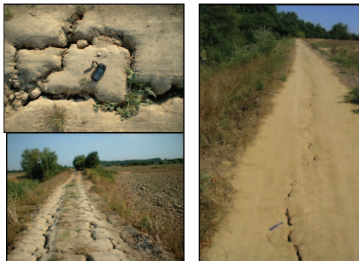
Figure 9. Fissures de dessiccation (Salmi ISL 2004)
