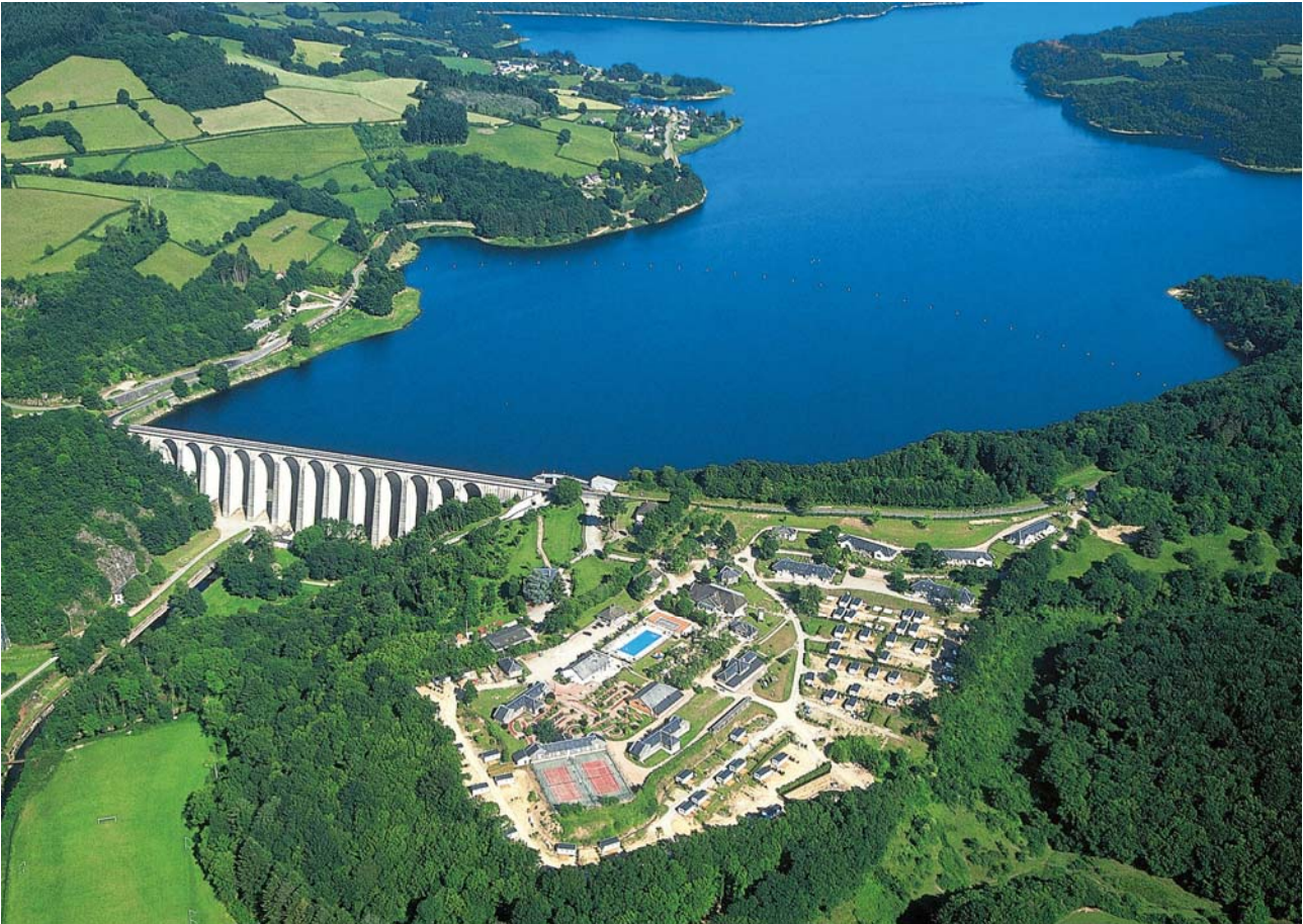
Figure 44: Aerial view of the Pannecière lake and dam on the River Yonne (Credits: Office de tourisme de France)
