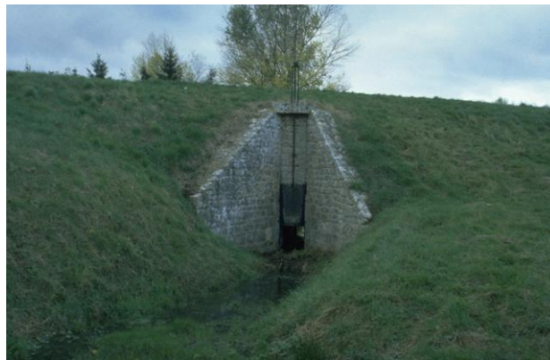
Figure 68: Photograph of Inlet Work on Gallery Land Side (with Flashboard Gate that May Be Operated from the Levee)
