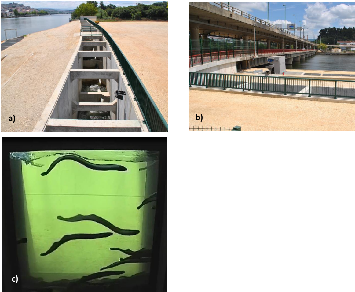
Figure 4.17. Fishway in Açude-Ponte Coimbra dam, River Mondego, Portugal. a) and b) lateral and upside views; c) lampreys passing through the window of the monitoring room (Photos: Pedro R. Almeida).
