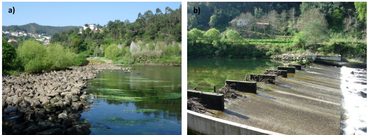
Figure 4.18. Two of the weirs located upstream of Açude-Ponte Coimbra dam that are being modified in order to build nature-like fish passages: a) Penacova and b) Louredo weirs (Photos: Pedro R. Almeida).
