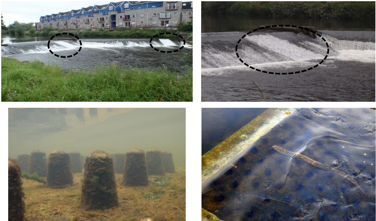
Figure 4.20. Plastic sheeting moulded to the form of egg-boxes placed in Annacotty weir, River Mulkear.
