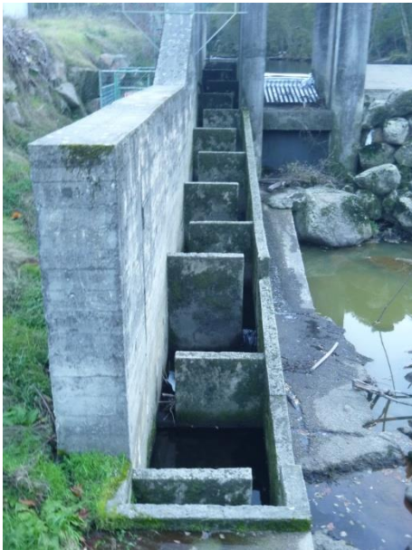
Figure 4.32. Example of two inoperable fishways in river Vouga, a Portuguese river basin where both lampreys and shads occur (Photos: Carlos Alexandre).
