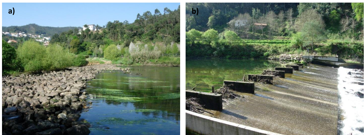
Figure 4.18. Two of the weirs located upstream of Açude-Ponte Coimbra dam that are being modified in order to build nature-like fish passages: a) Penacova and b) Louredo weirs (Photos: Pedro R. Almeida).
