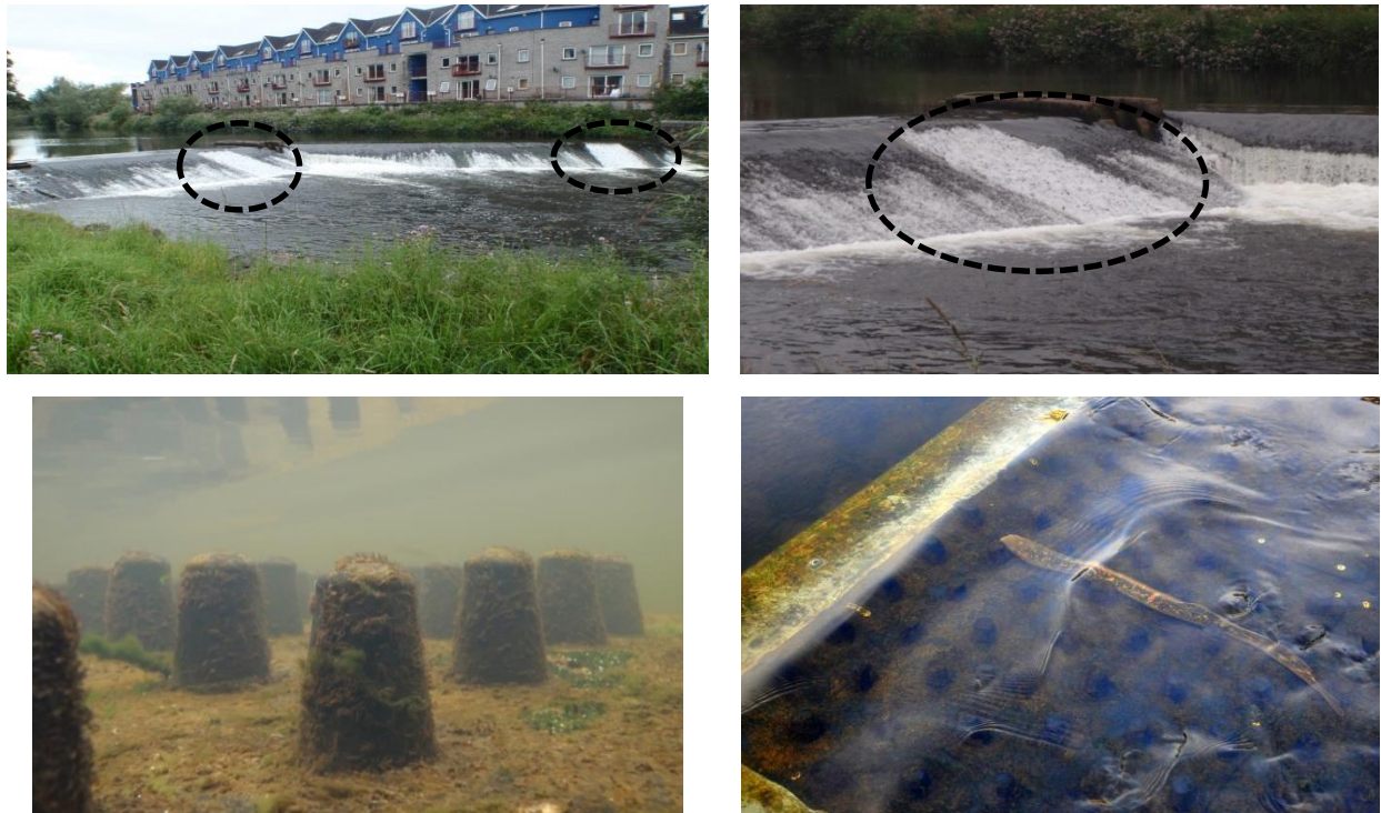
Figure 4.20. Plastic sheeting moulded to the form of egg-boxes placed in Annacotty weir, River Mulkear.
