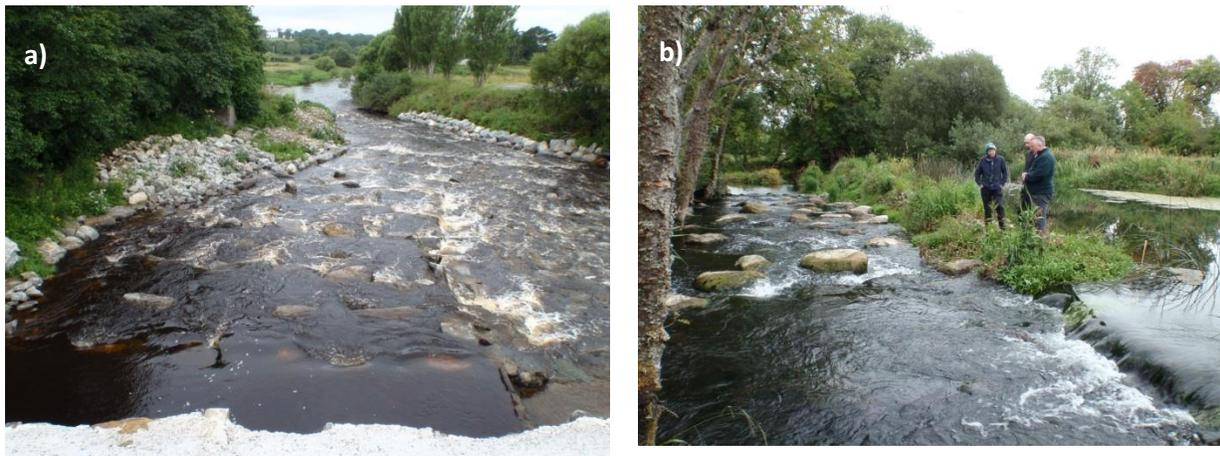
**Figure 4.21. Rock ramps installed in a) Abbeyfeale, Feale catchment. Feale is a salmon and sea lamprey catchment under Habitats Directive, and b) King's River, Nore catchment.**
