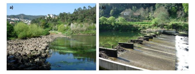
Figure 4.18. Two of the weirs located upstream of Açude-Ponte Coimbra dam that are being modified in order to build nature-like fish passages: a) Penacova and b) Louredo weirs (Photos: Pedro R. Almeida).
