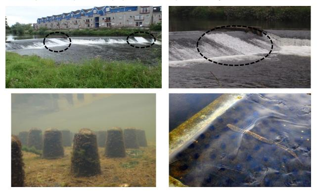
Figure 4.20. Plastic sheeting moulded to the form of egg-boxes placed in Annacotty weir, River Mulkear.
