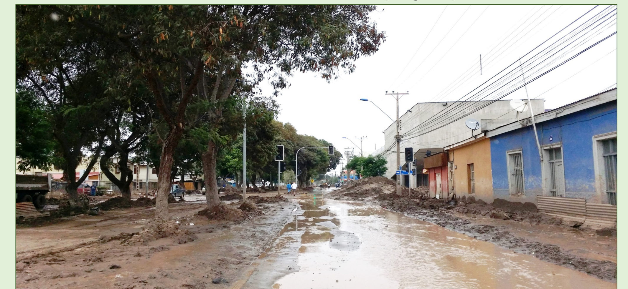
Fig. 5: Copiapó's street after the landslides
