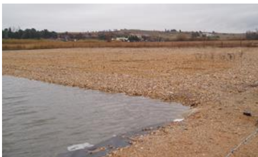
Figure 29 : Rockfilter de la station de Lespignan (source : SATESE 34)
