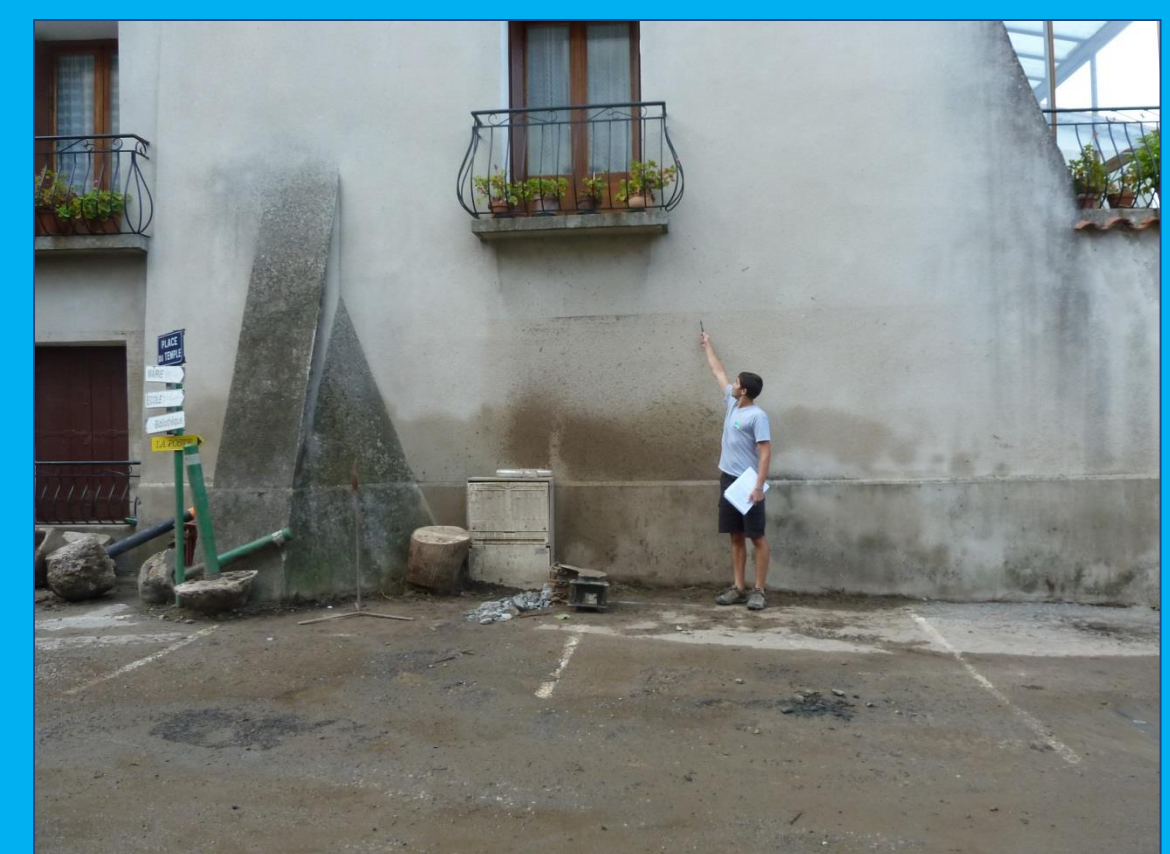
Witness mark of the flood of September 19-20, 2014, in Saint-Laurent-le-Minier (Hérault) - Source : C. Saint-Martin (Irstea, 2015)
