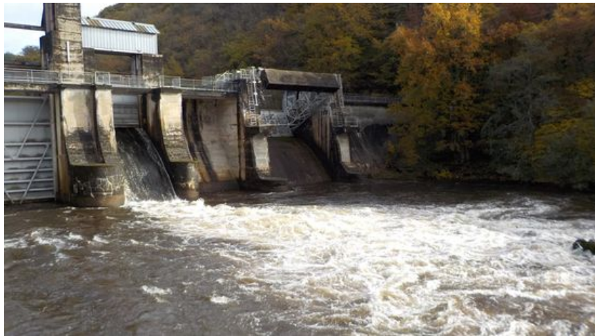
Figure 2.11: Discharge released by dam spillway (session # 3) (Source: A. Despax).
