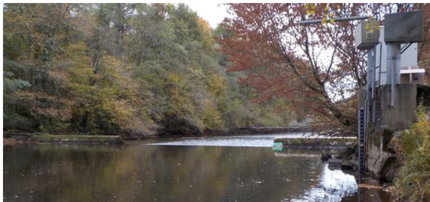
Figure 2.12: EDF-DTG hydrometric station with VEGA radar gauge (Source: A. Despax).
