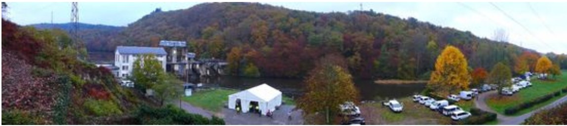
Figure 2.4: View of site, Chauvan Dam, the tent, the car park and Taurion River (Source: N. Everard, UK Environment Agency).
