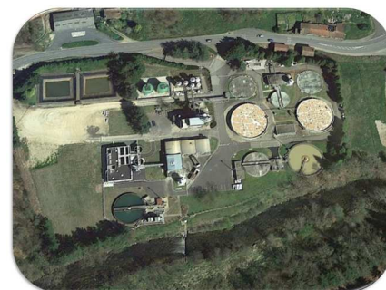
Sanofi Wastewater Treatment Unit
