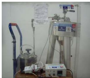
FIGURE 1. Thermal hydrolysis plant.
