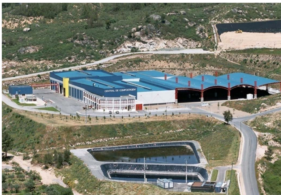
FIGURE 1 Resiestrela’s Composting Plant, sanitary landfill and WWTP.
