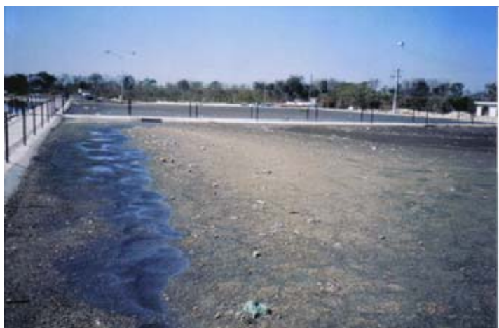
FIGURE 1 Oxidation ponds system in Mérida, Mexico.
