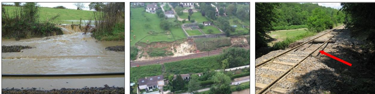
79 80 Figure 2: Illustration of surface runoff impacts on railways: from left to right, flood, landslide, and 81 breach in the embankment
