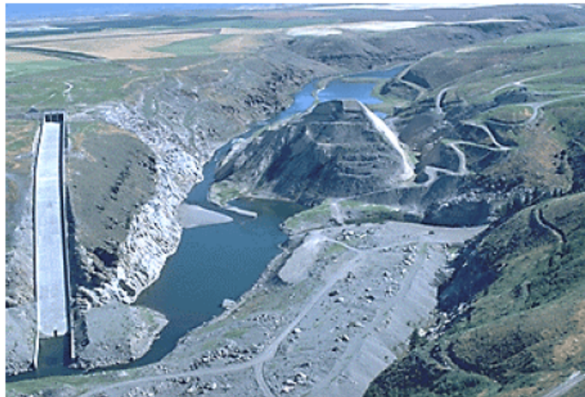
...and after failure
