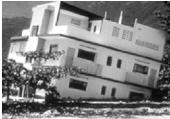
A partially sunken house illustrates the challenge of understanding how grains of soil interact with each other and under what conditions they will support structures.
