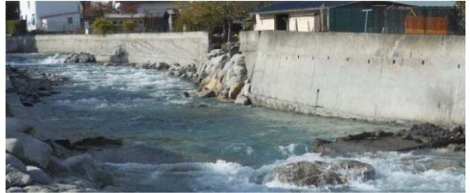
FIGURE 7 - RUPTURE ET REPARATION D'URGENCE D'UNE DIGUE - GAVE DE CAUTERETS - PIERREFITTE (65) - 2013 (ONF-RTM)
