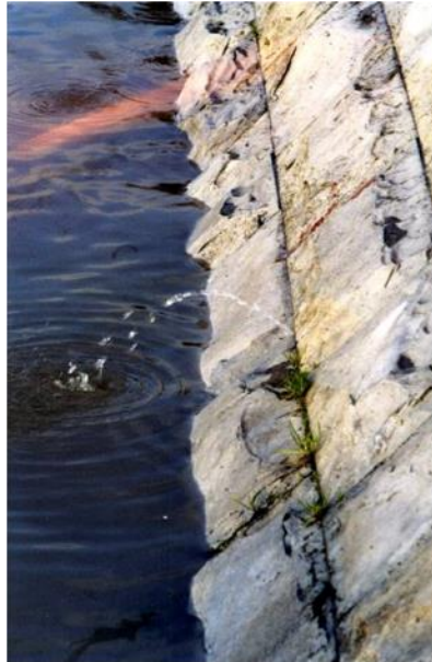
Figure F-6: Post flood inspection finding evidence of leakage in the masonry revetment, probably involving an important void behind the revetment, filled with water during the flood (source: Rémy Tourment)
