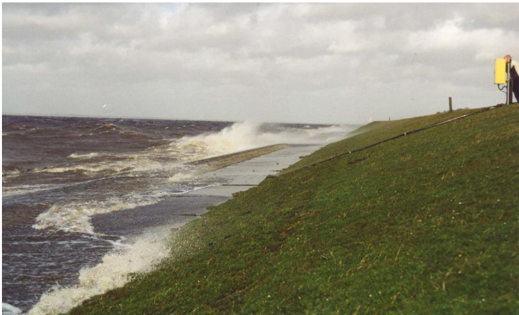
Figure NL-1: Rural lake-side levee during storm, with waves well above 1 metre (rubble-stone waterline berm and lower half of slope with placed stone partly submerged).
