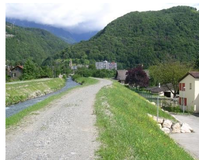
A torrent levee in Domène
