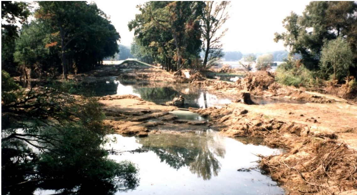
Figure D-4 Levee Failure at the Oder 1997 near the village Wiesenau. Foreground: large scourholes in the levee axis. Background: remaining levee cross section. Trees at the landside toe hindered the levee slope inspection. On the right side: the Oder river. (photograph: R. Pohl)
