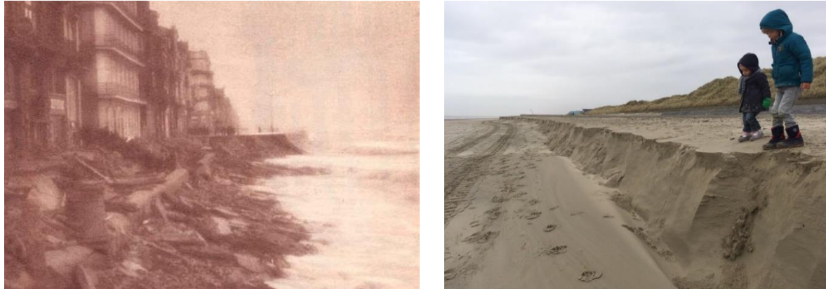
Figure B-8. Near failure of the Belgium coastal defence at Knokke-Heist in 1953 (Source: Le Patriote Illustré) and, more recent, formation of cliffs in 2013 (Source: T. Verwaest)
