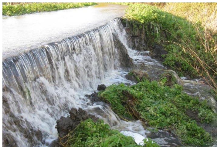
Figure B-14. Headcut formation following a low-head overflow event along the Durme in 2010 (Source: FHR)
