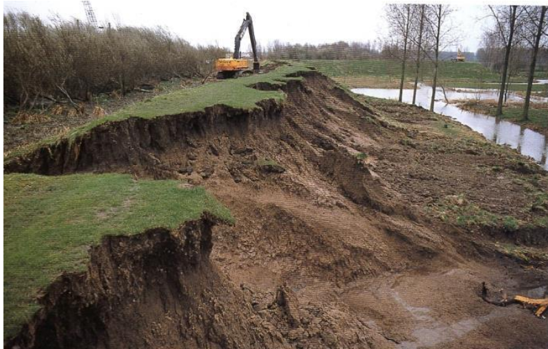
Figure B-10. Failure of the land-side slope along the Sea Scheldt in 1990 following overtopping (Source: A. Van Hoyweghen)
