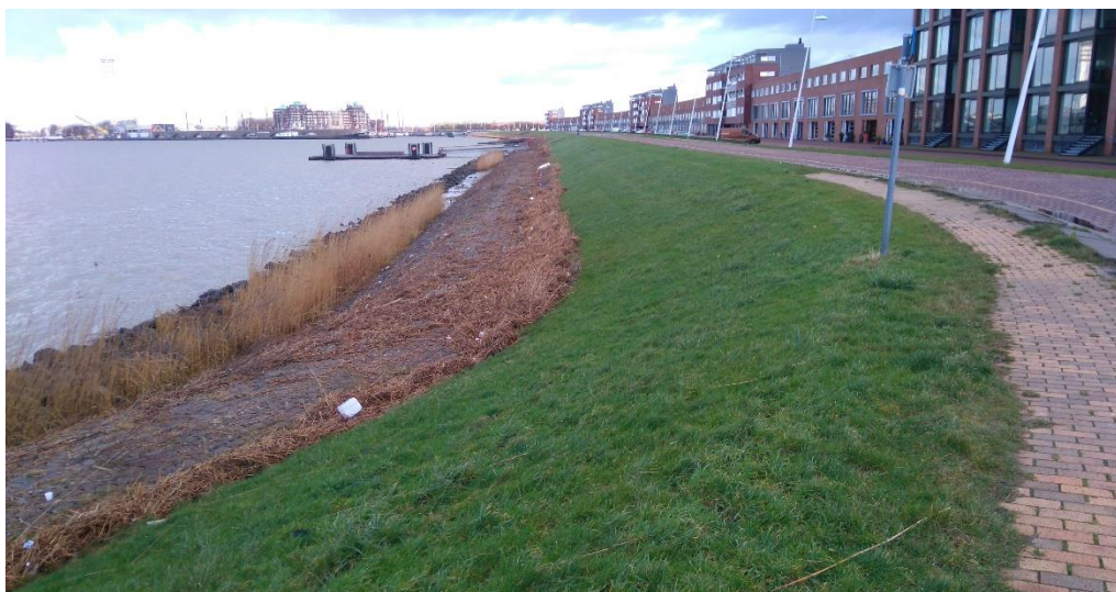
Figure NL-2: Broad urban levee in Lelystad with flotsam from recent storm (offshore breakwater sheltering the levee not visible).
