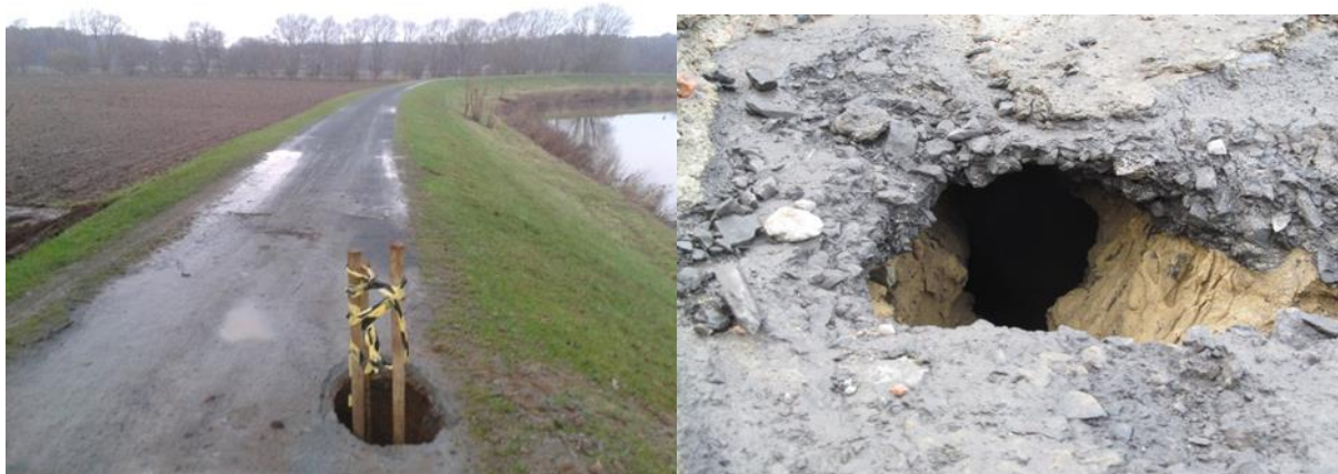
Figure B-16. Animal activity discovered by coincidence (Source: de Vlaamse Waterweg nv/FHR)
