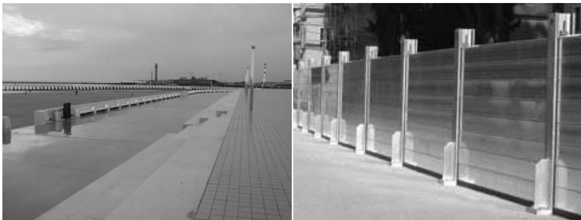
Figure B-4. Flood defence measures along the Belgian Coast (Source: Coastal Division)
