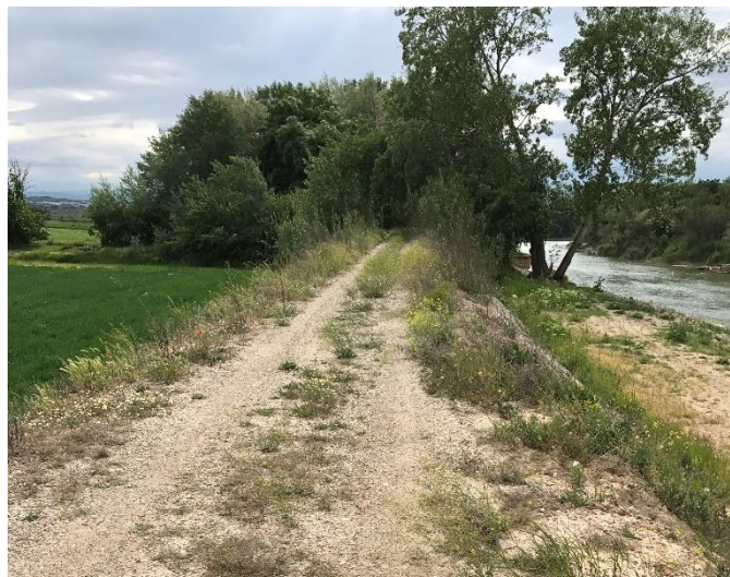
Figure ES-2. Levee segment in the Ebro river in Novillas (Zaragoza). Source: MITECO (Spanish Ministry for Ecological Transition).
