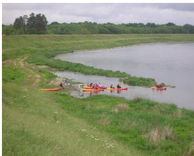
A fluvial levee near Orléans
