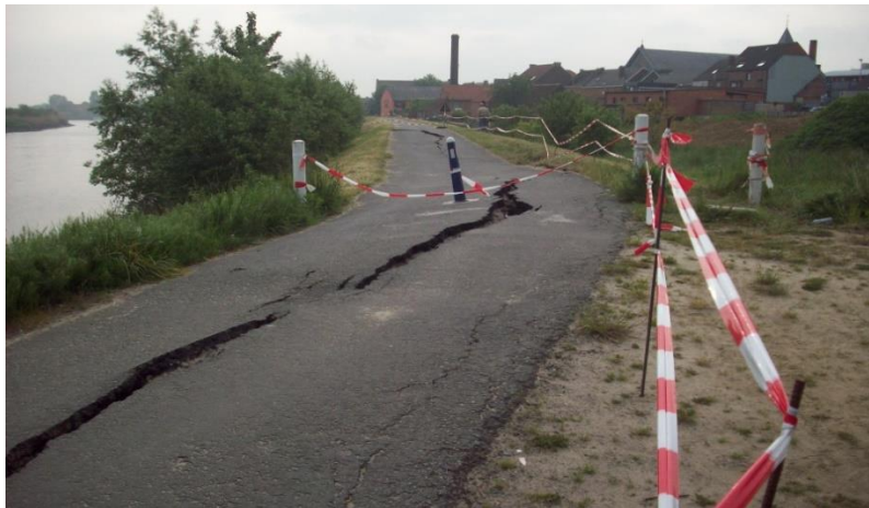
Figure B-13. Slope instability in Schoonaarde along the Schelde (Source: De Vlaamse Waterweg nv)
