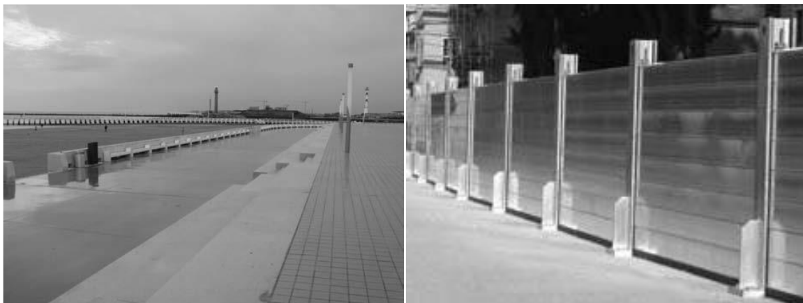
Figure B-4. Flood defence measures along the Belgian Coast (Source: Coastal Division)
