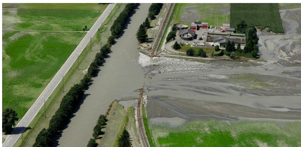
Figure CH-11: Levee breach at river Aare near Meiringen (BE), August 2005 (© Swiss Airforce).
