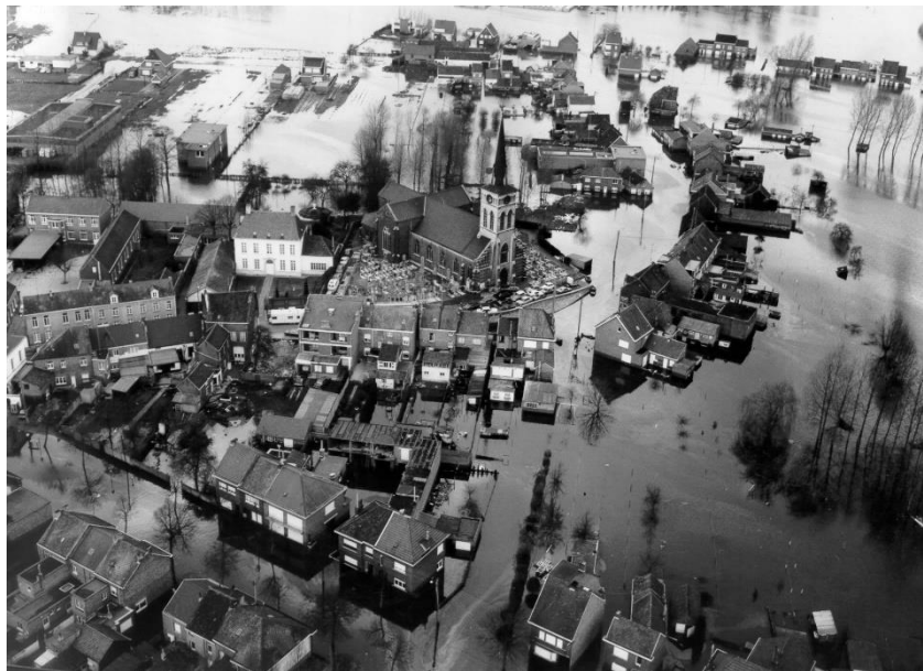
Figure B-9. Flooding of village of Ruisbroek in 1976 (Source: FHR)
