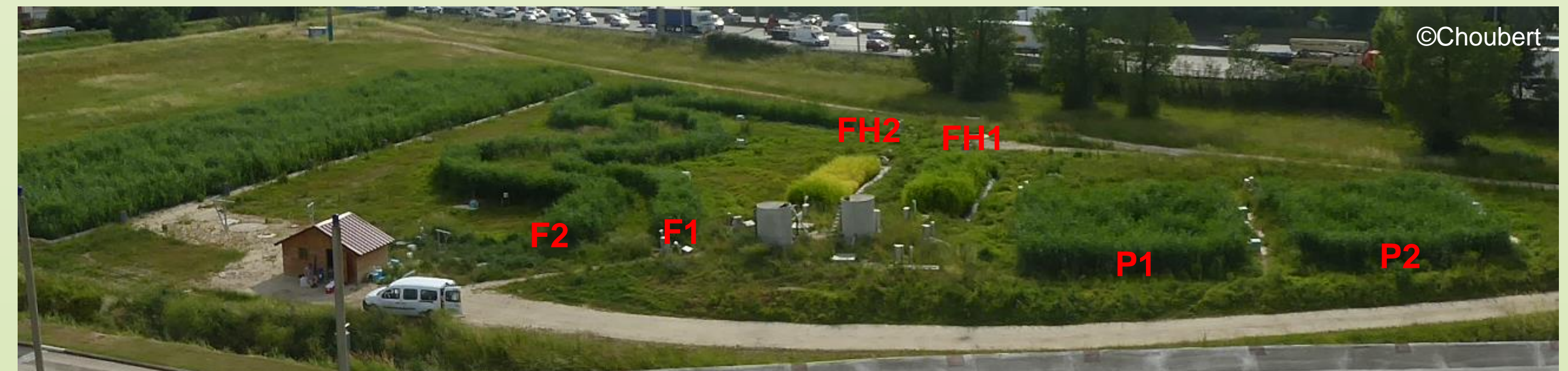
Fig. 6. CWtw with different configurations (meadows, ditches built with soil and adsorbing materials) studied during the BIOTRYTIS project
