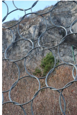
Figure 1: 4-contacts ring net [Coulibaly et al., 2017b].
