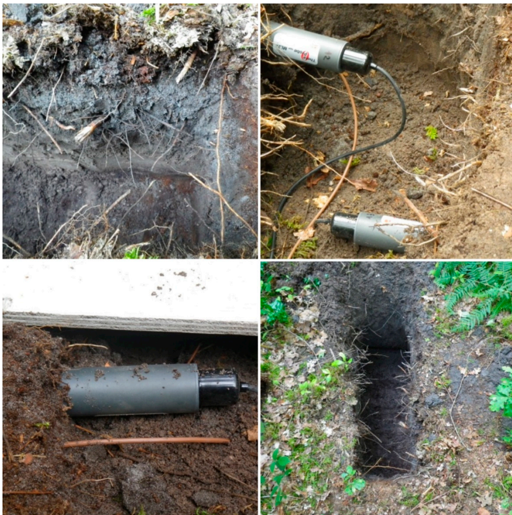
Figure 2. Installation of the soil moisture sensors at FRAYE site.
