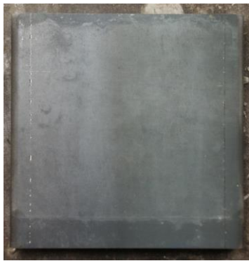
85 86 87 88 89 90 Fig. 2: New formwork surface
