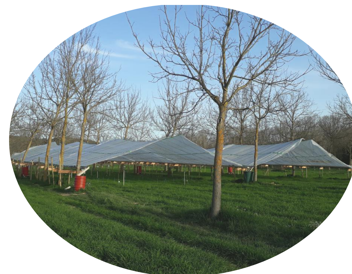
Cable structure with folding tarpaulins. Covers 2 alleys (over ~800 m 2 ).
