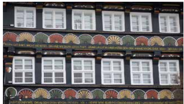
Half-timbered building in Osterwieck (photo: S. Neumeier)
