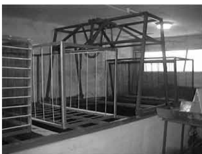
Tanks, cages and cranes used in the soaking and pasteurization process
