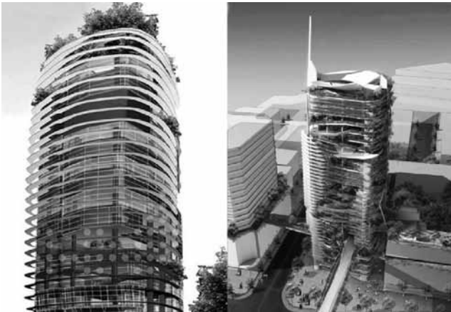
Image 1, Hamzah & Yeang Architects
