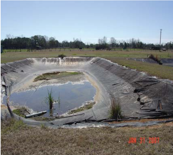
A pond at the start of the project
