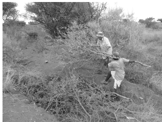
Figure 1 Branches of A. mellifera packed in a gully head to form a filter.
