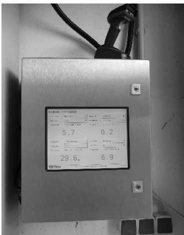
Figure 1. TENferm central unit with the touch-monitor displaying actual results on a biogas plant
