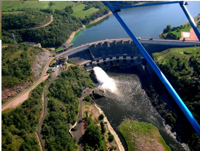
Villerest dam (France)
