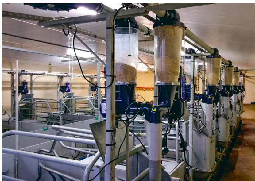
Photo 5. General view of one lactation room with two feed dispensers per pen.
