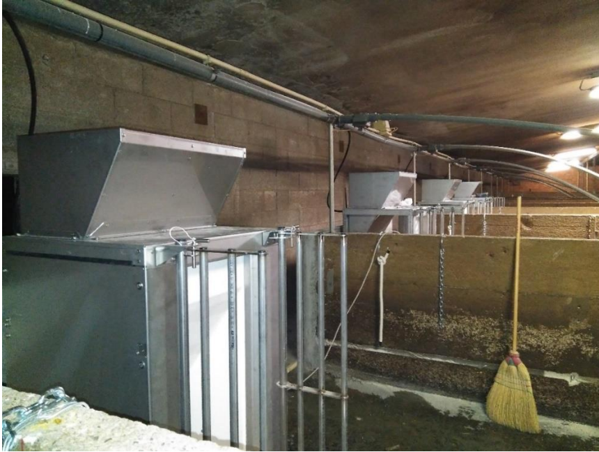
Four stainless individual precision feeders were installed in Italy.
