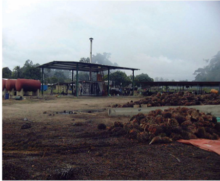
Figure 6 (S. Rafflegeau): Examples of investment in the mini-mill, a semi-industrial extraction unit by managerial enterprises of producers: Global view of a container extraction unit processing stemmed fruit in Côte d'Ivoire.
