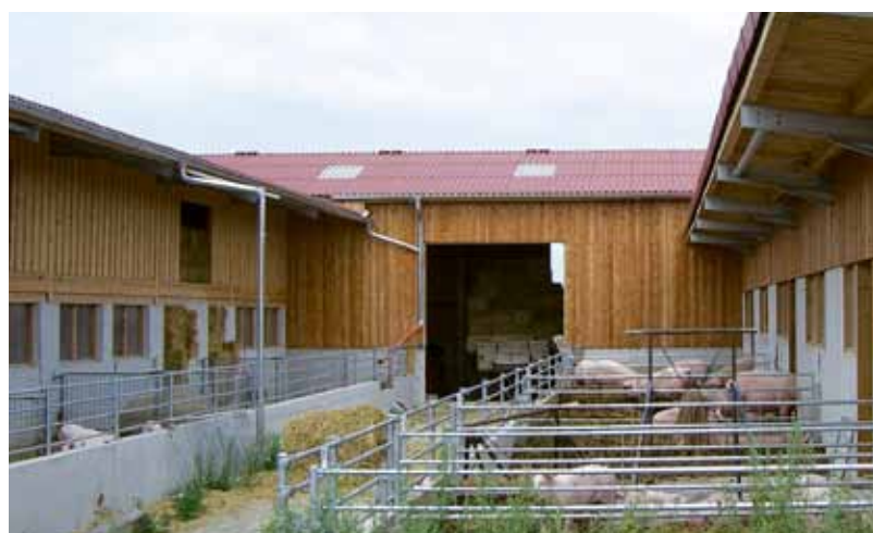
Indoor housing systems in organic farming must provide an outdoor run, so the pigs can experience climatic influences of sun, rain and wind.
