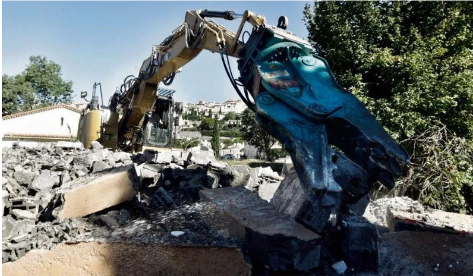
Figure 56 : Removing houses located in the Brague high flood risk area has yet started (source: Nice-Matin, © Frantz Bouton, https://nouveau.pressedd.fr , published on Oct. 3 rd , 2018).
