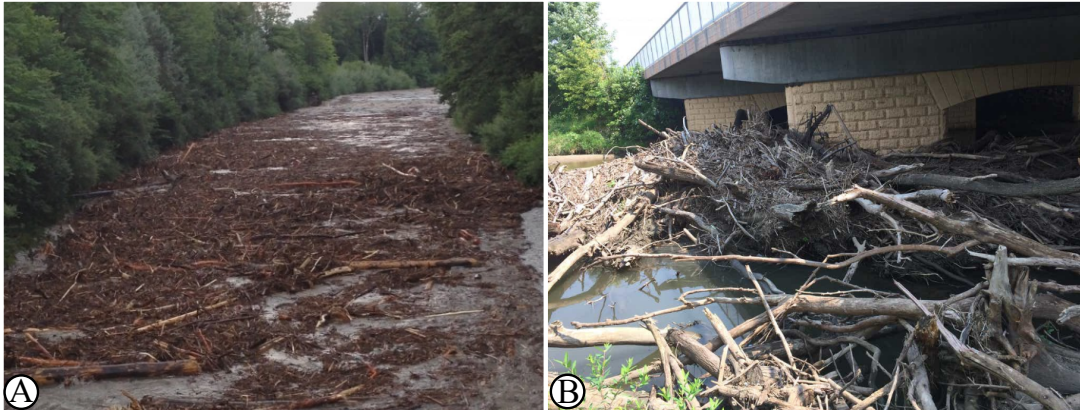
FIGURE 1.3. (a) LW transport (source: https://energisch.ch/ ); (b) LW accumulation at a bridge (source: https://eu.desmoinesregister.com/ )
