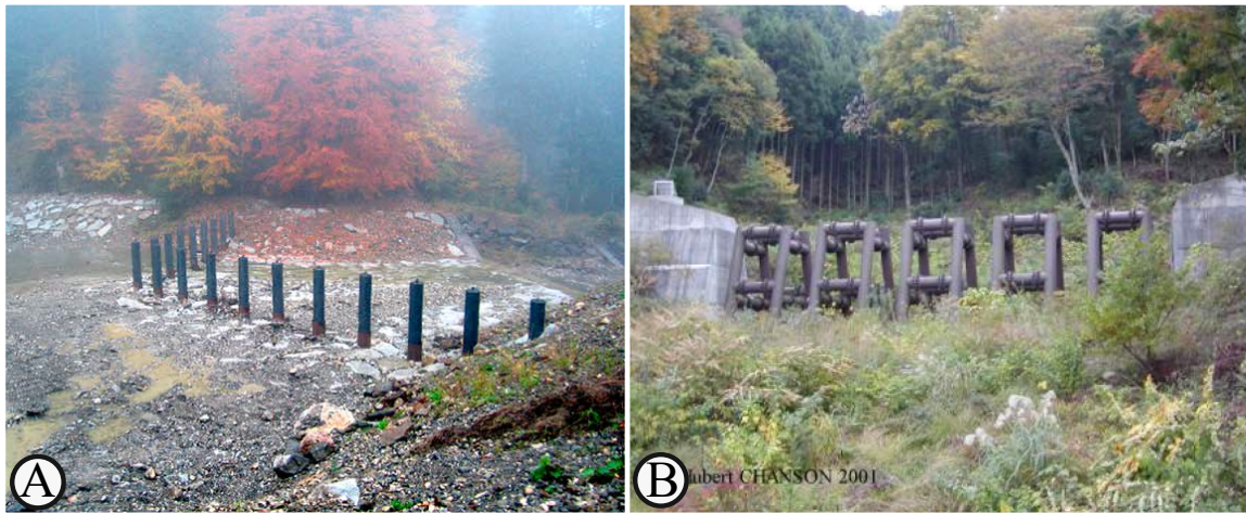
FIGURE 2.1. Light structures: (a) V-shape sectional dam made with piles (Ruiz-Villanueva et al., 2016b); (b) SABO dam tubular (Chanson, 2004b)
