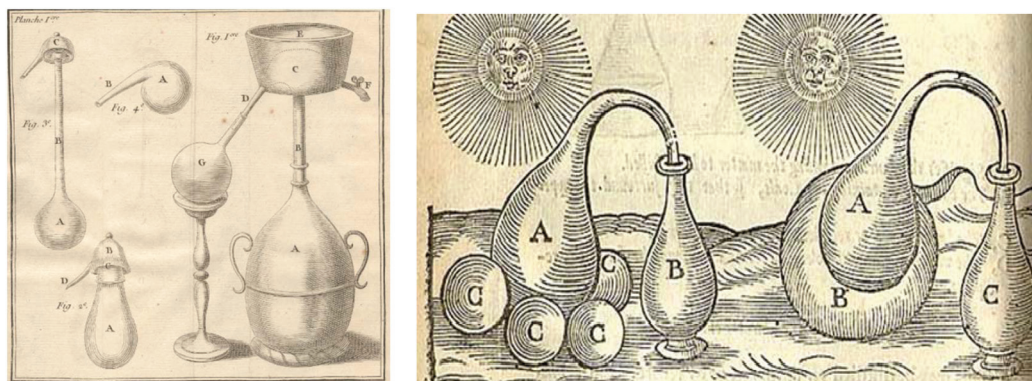
Fig. 1 Innovative alembics by Macquer (1756) 2 and French (1651). 3
