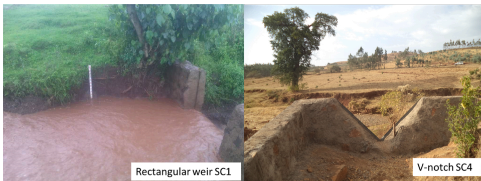
Fig. 3. Setup of weirs and diver/staff gauge at the outlet of the sub-catchments.
