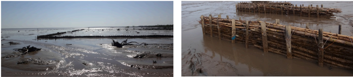
Fig. 11. Permeable dams constructed near Weg naar Zee, north of Paramaribo, Suriname (photos by E. Van Lavieren).
