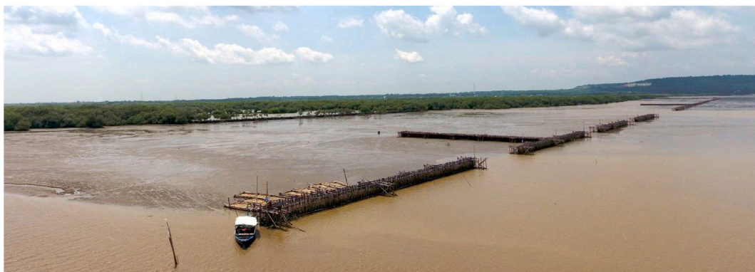
Fig. 8. Example of permeable dams in Gresik Regency, close to Solo River, Java, Indonesia (photo by MMAF early 2019).
