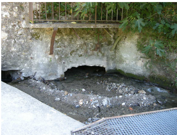
(a) Canal Saint-Hippolyte (Gard)
