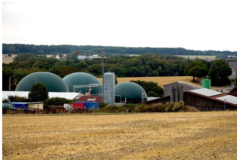
Figure 22: Biogas Plant Karle / Agro Energie Hohenlohe GmbH & Co. KG; blue containers in from: pilot plant for nutrient recovery (picture credit: IBBK Fachgruppe Biogas GmbH)
