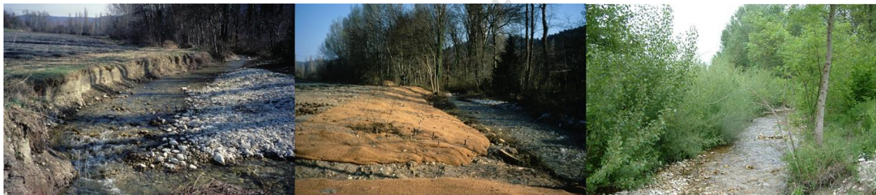
Figure 4. Photo of a riverbank soil bioengineering work before, during and four years after the implementation
