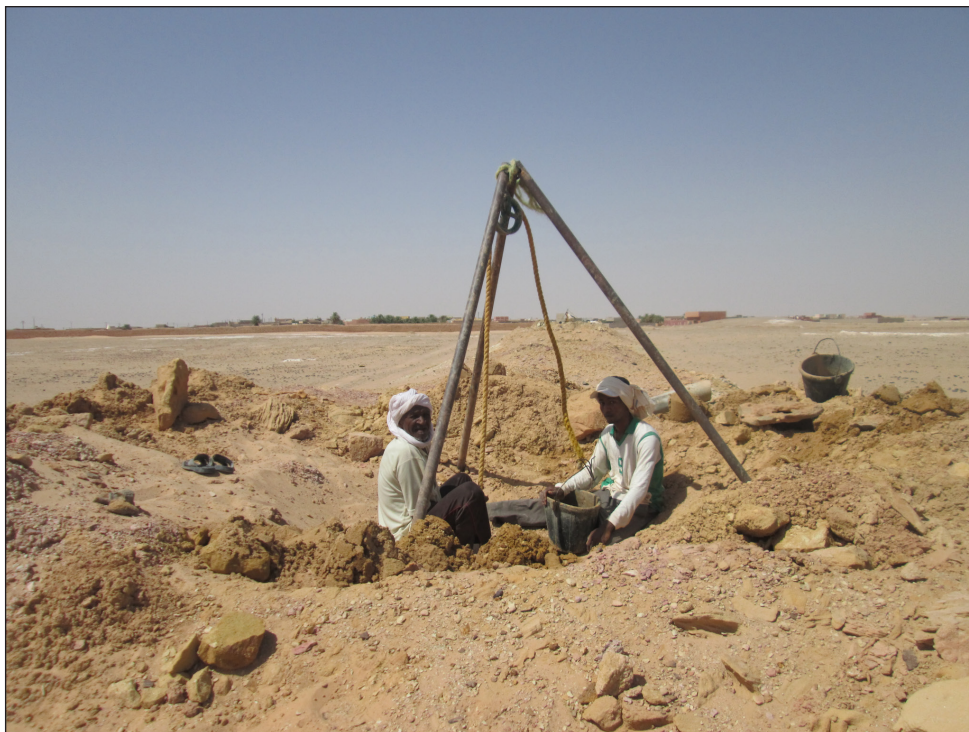
Picture 1 Two young men (one inside the well, not visible in the photo), accompanied by an elder, on duty maintaining a well (August 2016).
