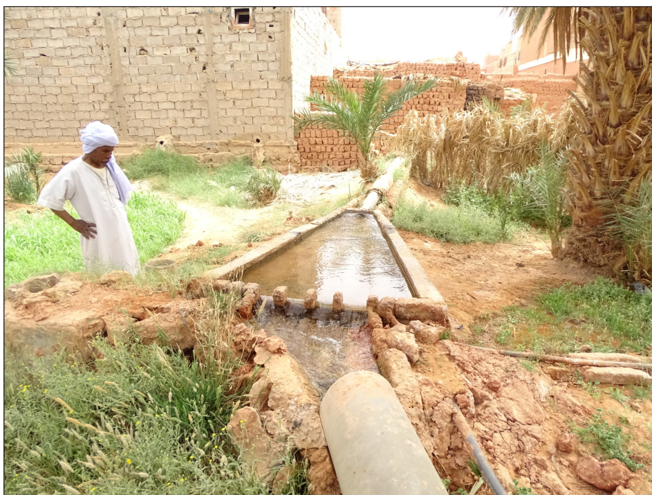
Picture 3 Replacing traditional channels by modern pipes while keeping the use of the water sharing basin ( kesria ) to ensure the visibility of water distribution for all. On the picture, the channel upstream of the kesria (top of the picture) has been replaced by a concrete pipe carrying all of the discharge of the foggara. In the kesria , part of the foggara discharge is diverted to smaller pipes that go left and right on the picture. What is remaining is the combined discharge of several water owners that will be transported in the big concrete pipe further downstream, where there is another kesria to sub-divide between these owners. (April 2017).
