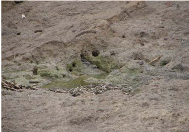
Figure 3.11 View of animal burrows beneath water side mid-slope of breach section (22 July 2008).
