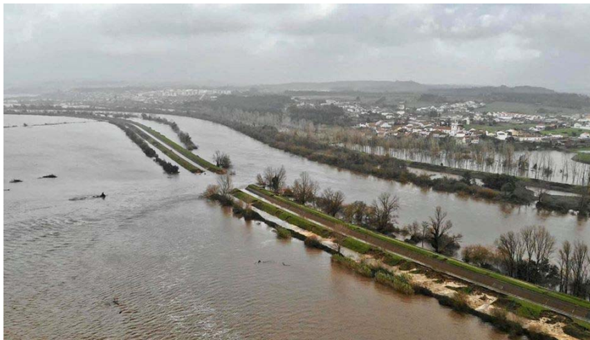
Figure 3.21 View of Santo Varão after collapse of the embankment 5 .
