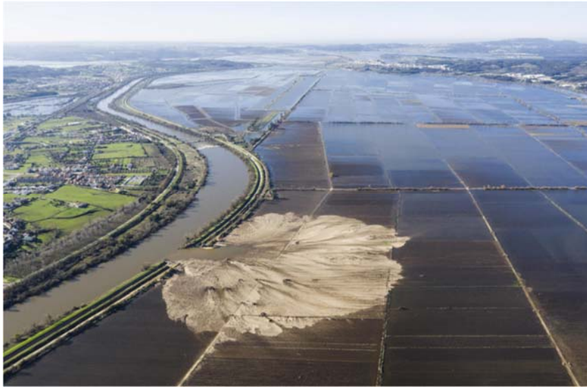
Figure 3.20 View of Santo Varão shortly after collapse of the embankment 4 .
