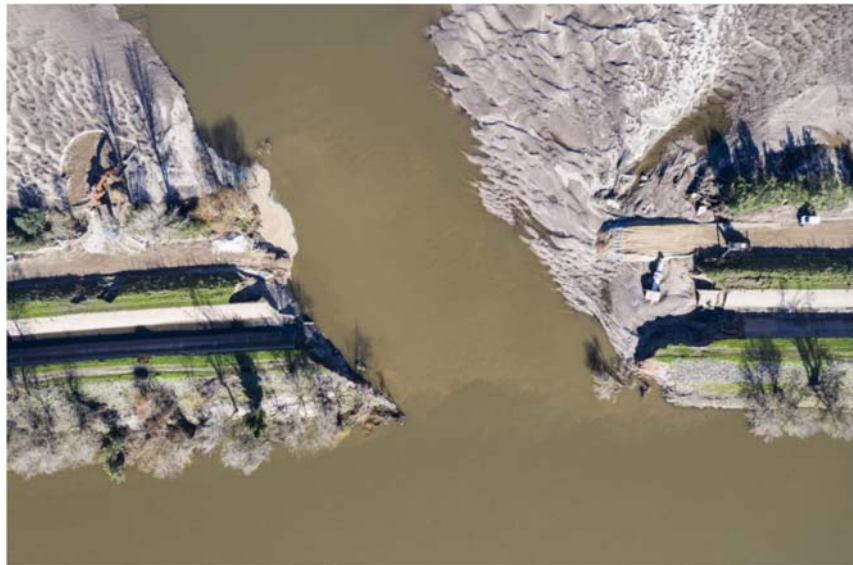
Figure 3.22 Top view of collapsed embankment in Santo Varão 6 .
