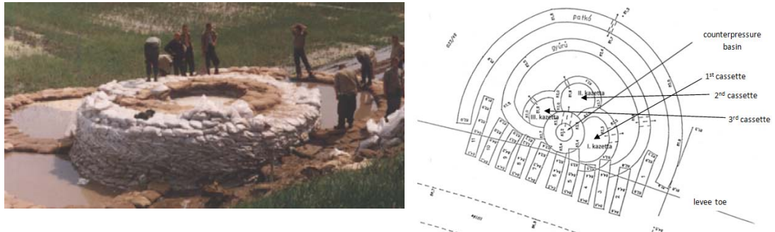
Figure 3.39 Counterpressure basin for related cassettes (left) and location of sand cassettes (right).
