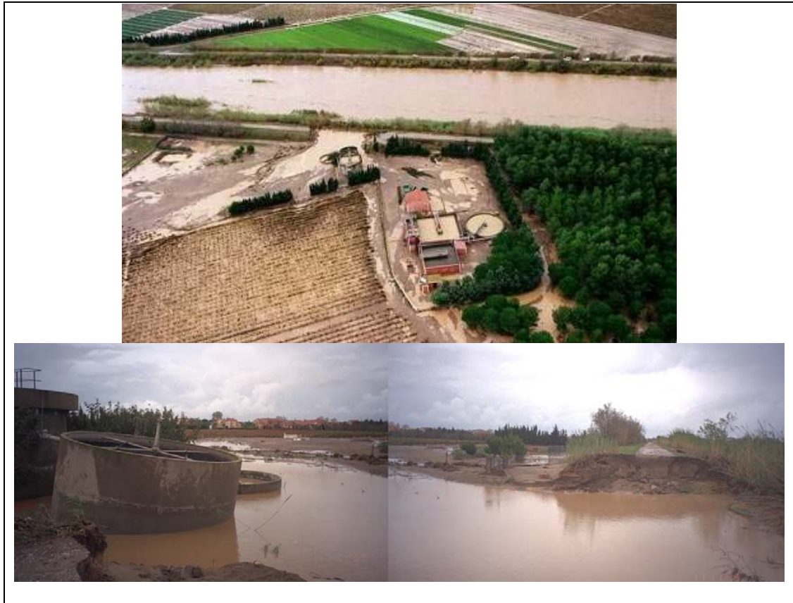
Figure 3.49 Breach in 1999 at St-Laurent-de-la-Salanque.
