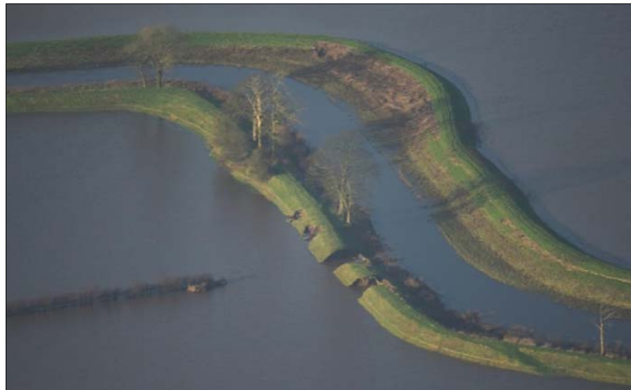
Figure 3.2 Photograph of the situation.
