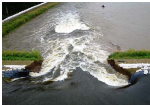
Figure 3.10 Breach occurring (taken around 0700 hr, 27 June 2008).
