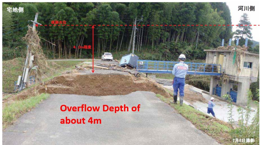
Figure 3.32 Picture of overtopping from the presentation 'Picture-Card Show Project' in JGS-JCES', contribution by K. Maeda, M. Ishihara and H. Mori, using materials from the Ministry of Land, Infrastructure, Transport and Tourism in Japan.
